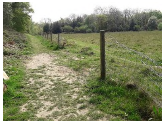
Broken fence in Dell Field
