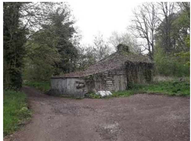
The Pump House
