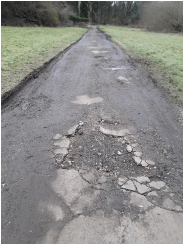
Surfacing of track along Footpath 02
